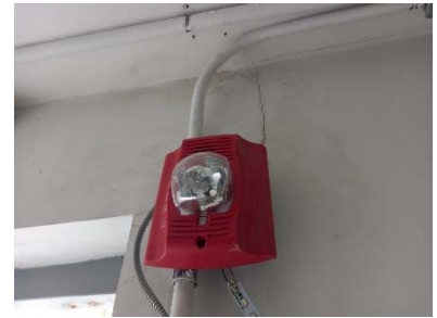
Fire Alarm Horn Strobe
