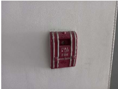
Fire Alarm Manual Station
